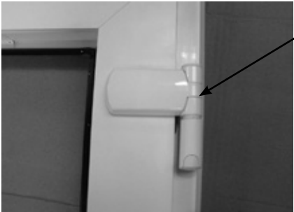
To adjust the door vent horizontally (left to right). Open the door and push in the plastic clip.
