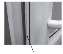
Adjusting the hinge as shown will correct this clearance.
