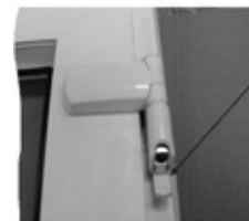
Adjusting the hinge as shown will correct this clearance.
