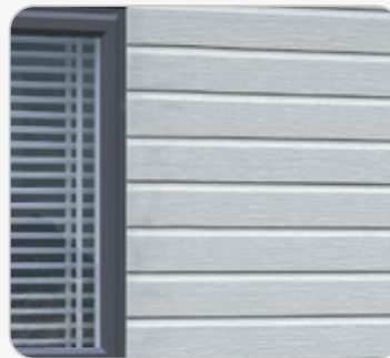
BONDED EXTERIOR WALLS 'Sandwich' construction walls provide a more rigid exterior, bonded with insulation in the middle
